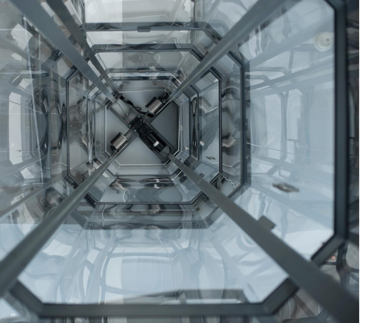
Vuelift® elevators are driven by an energy-efficient winding-drum drive train system, using two military-grade aircraft cables for a smooth and stable ride.
